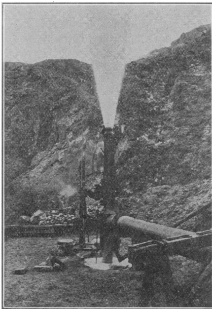
A "gusher" of steam instead of oil. The slender instrument alongside measures the pressure by means of a column of mercury.
