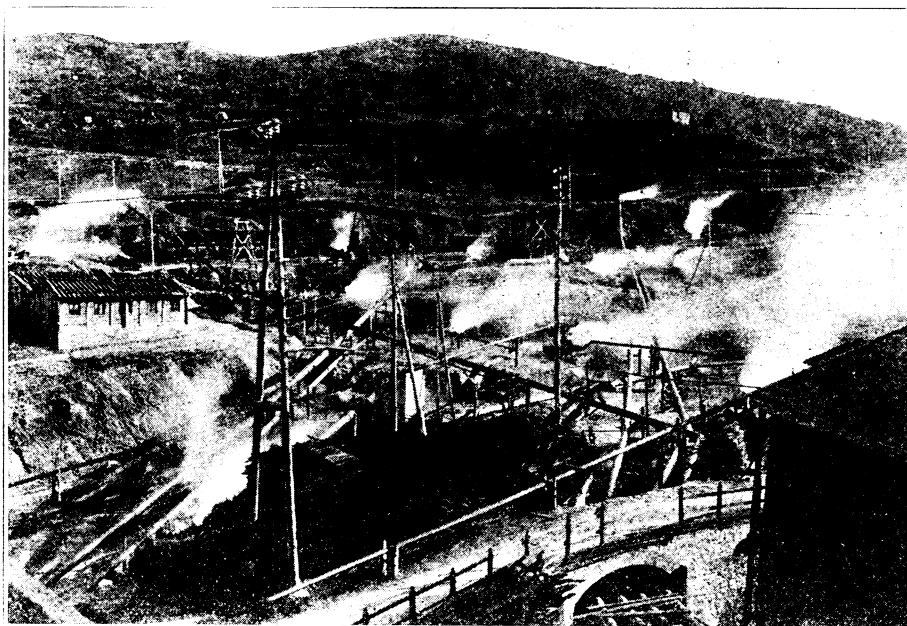
View across the valley at Larderello, in Tuscany, Italy, showing the webwork of steam pipes and high-tension electric wires that turn into useful power hitherto wasted energy—and steam, steam, everywhere.
