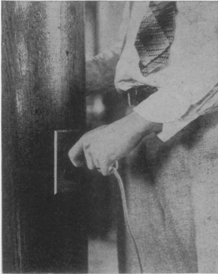
AN ELECTRIC PLUG waist-high that requires no gymnastics or stooping. Pulling the connection straight out is also found to be less of a strain on the wires, and lessens the chance of short-circuiting
