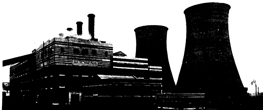
CONCRETE COOLING TOWERS AMERICA DOES NOT NEED These huge towers with an hourly circulation of 5,000,000 gallons cool condenser water at the modern Hams Hall generating station, Birmingham, England. In this country it is usually possible to build power plants near streams where a continuous supply of cool water is available.
