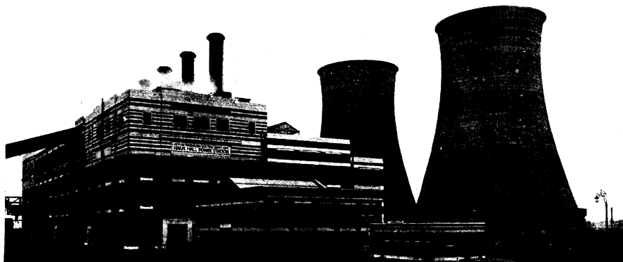
CONCRETE COOLING TOWERS AMERICA DOES NOT NEED These huge towers with an hourly circulation of 5,000,000 gallons cool condenser water at the modern Hams Hall generating station, Birmingham, England. In this country it is usually possible to build power plants near streams where a continuous supply of cool water is available.
