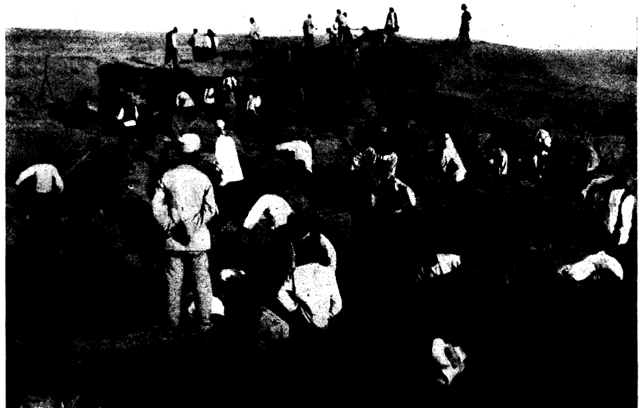
DIGGERS AT WORK
