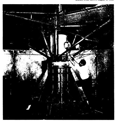
WHIRLING ARM FOR AIRSHIP TESTS
