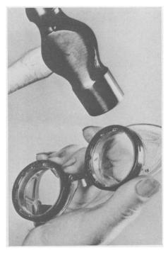
These are goggles that really protect the eyes against flying missiles, hot sparks, even a light blow with a hammer. They are made of a tough transparent plastic which though clear as crystal, oddly enough is made from coal and petroleum.
