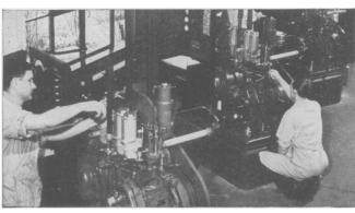
**CLUE No. 6...** The final clue is an easy one—if you're an automotive or petroleum engineer. These machines are "C.F.R." knock rating engines which are used in the six gasoline-testing laboratories.
