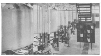
**CLUE No. 3**...Tons of the various ingredients that make the finished product are blended in these weigh tanks at one time. They measure the ingredients accurately to within one part in ten thousand.
