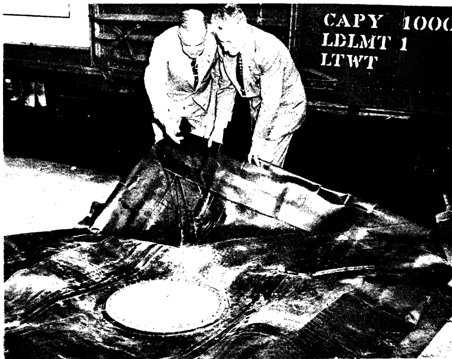
SYNTHETIC RUBBER BAGS that can convert ordinary steel boxcars into gasoline carriers, were recently given their first demonstration in Washington, D. C. Here one of them is being examined by J. B. Eastman, Director of Defense Transportation (left) and Reid Gray, inventor of the device.
