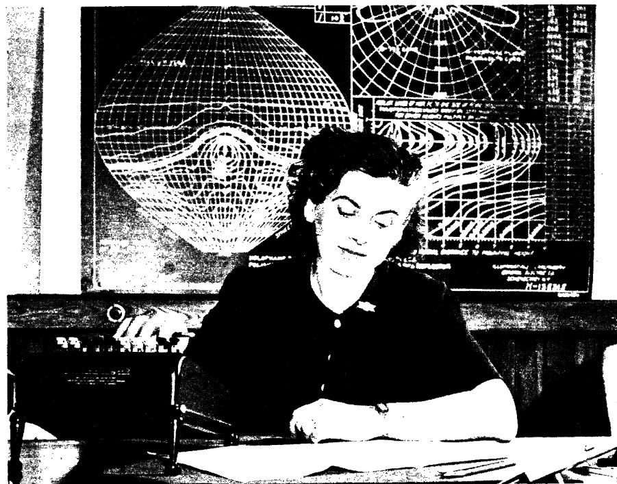
CURVES, isocandle and isolux, are being computed by Miss Ruth Forbes of General Electric. In the background are charts showing the lines which indicate distribution of candle power from a light unit.
