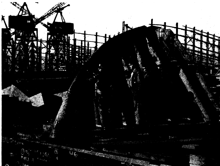
PRE-FABRICATION —To speed the flow of ships off the shipways, whole sections of the hull are now assembled before they are lifted into place. This is an official U. S. Maritime Commission photograph.
