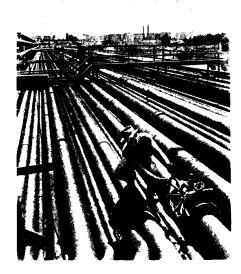
SEGREGATION — Through many miles of pipes like these, crude oils are segregated. The operator in the foreground is opening a valve to let a certain batch of crude flow to its destination at a Standard Oil Company (New Jersey) refinery.
