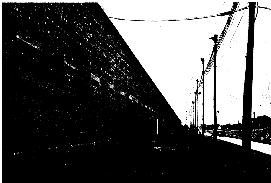
FACTORY FINISHED —The walls of this built-from-the-top factory, and the concrete floors laid directly on the ground without steel reinforcing, are now finished. Machinery has been moved into the first section, and production is booming, while the other sections are being constructed.
