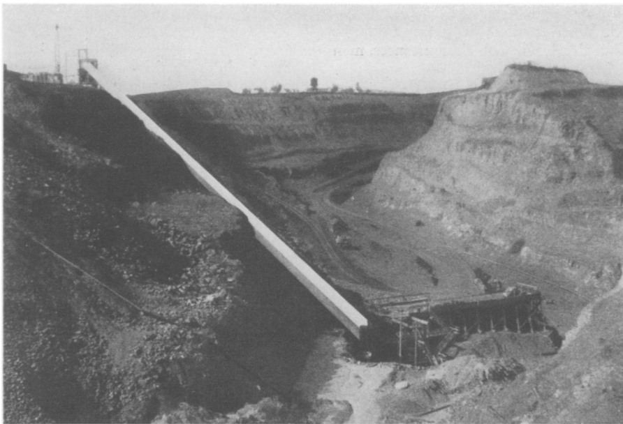
CARRYING ORE —The nation's first steel-carriage conveyor belt, developed by the Goodyear Tire and Rubber Co., is used to speed iron ore up the 1,100 foot slope from the open pit mines of the Oliver Iron Mining Company, near Hibbing, Minn.
