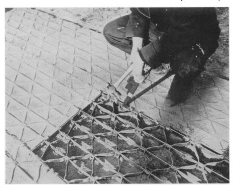
PORTABLE ROADBED—This modern variation of the old dirt road shows post-war promise, especially where a practical roadbed must be quickly laid for temporary use, such as detours. The air forces now use it to make portable emergency landing fields. The steel grating panels are easily connected with hammer and pronged tool. Then sand is filled in between meshes.
