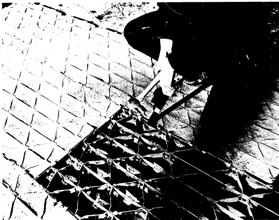
PORTABLE ROADBED —This modern variation of the old dirt road shows post-war promise, especially where a practical roadbed must be quickly laid for temporary use, such as detours. The air forces now use it to make portable emergency landing fields. The steel grating panels are easily connected with hammer and pronged tool. Then sand is filled in between meshes.
