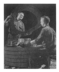
THIN STEEL—Heart of an escort ship's electric drive is this rotor core for a motor under construction for the U. S. Navy at the Westinghouse East Pittsburgh Works. It is composed of hundreds of hoop-like sheets such as this, each about one-fourth as thick as a dime. The "teeth" form slots into which copper coils are inserted.
