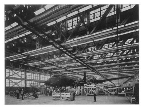
NEW PLANT—A big Douglas C-54 cargo transport is shown being finnished just inside the door of the new all-timber assembly plant just constructed at Chicago by the Austin Company. By use of laminated timber construction and in other ways, it is estimated that more than 30,000 tons of steel and important metals were saved in putting up this plant. Notice the great beams that look like steel girders.
