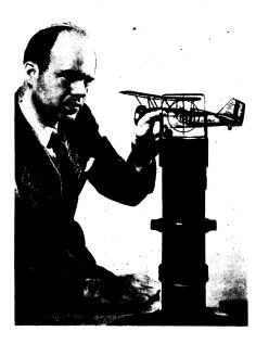
lenses and an unsilvered mirror through which the pilot looks. The picture shows one of the sights trained on the moving image of a plane in the background. The new sight duplicates performance of a combat sight at a tenth the cost.
