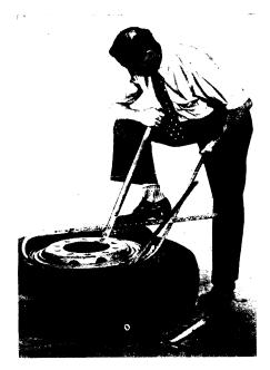
TIRE CHANGER—This new Firestone bead-loosening tool makes it easier to remove heavy truck and tractor tires stuck to their rims. One of the detachable hooks has been forced, by leverage, between the tire iron and the rim. This exerts tremendous downward pressure on the tire, forcing the bead away from the rim.
