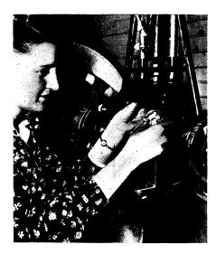
TESTING BOMB FUZE—A fuze for a 20-pound fragmentation bomb is being installed in the path of a man-made gale to determine how the fuze would perform when dropped by an American airman. Wind tunnel tests such as this at the Westinghouse East Springfield plant provide a constant check on the quality of fuzes produced.
