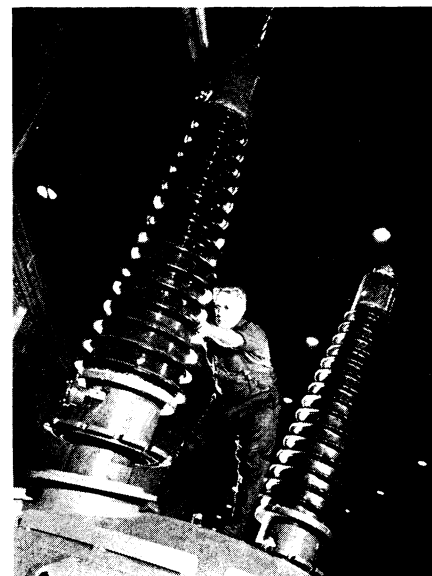
GIANT "SPARK PLUG" —This 14-foot condenser bushing is part of a huge automatic switch that will guard flow of electric power into a new Westinghouse war plant. The bushing conducts 230,000 volts of power into the tank on which the workman is standing, just as a spark plug in your automobile conducts electricity into the gas-filled cylinder.
