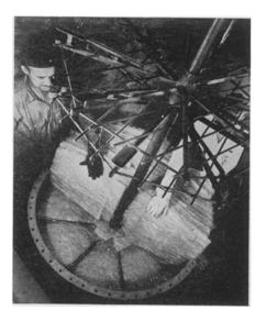
VERSATILE — Another use for glass, in the form of fibers 85/10,000 of an inch in diameter, is in the production of alcohol as packing for distillation columns, replacing critical materials. The picture shows the packing process at the Tom Moore Distillery, Bardstown, Ky. The glass fibers used are manufactured by the Owens-Corning Fiberglas Corpora-
