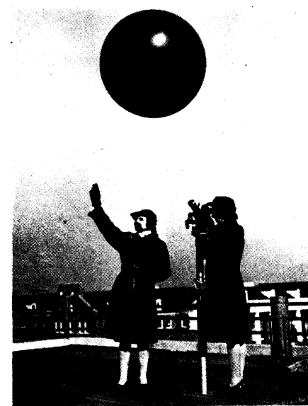
AIR WAVES —The part these two WAVES are playing, in manning the shore jobs so that men can be released for the fighting fronts, is a highly technical one. The aerographer's mate (left) is loosing a pilot balloon at the Naval Air Station, Anacostia, D. C., while the officer aerologist (right) prepares to follow the path of the balloon with a theodolite. Their study of atmospheric conditions is essential for maintenance of an air station. Official U. S. Navy photo.
