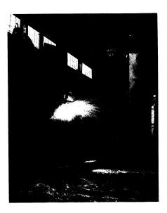
SPARK BARRAGE—This welder is using an oxy-acetylene torch to work on one of the big steam lines for Westinghouse roving Power Trains, which will be used to restore electric service in cities reconquered from the Axis by United Nations armies. Each eight-car train is capable of generating 5,000 kilowatts.
