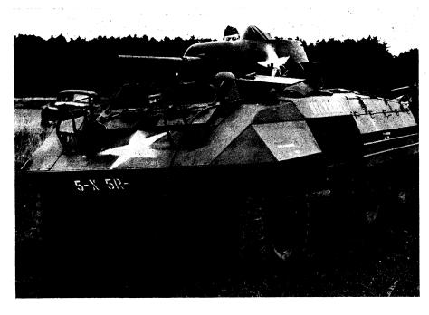
RECENT ADDITION—This is the eight-ton Armored Car M8, designed by the Ordnance Department to combine the speed and maneuverability of an automobile with the punch and armored protection of a light tank. It has a protectively low silhouette, resembling a turtle's back, and mounts both a 37 mm. cannon and .30 caliber machine gun. A crew of four handles this vehicle, which is intended primarily as a combat reconnaissance car. U. S. Army Signal Corps photograph.
