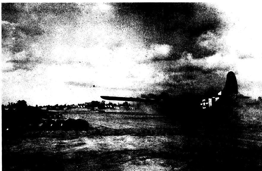
NO WAITING —Although only partially completed, this airfield somewhere in France is already in use for gliders loaded with supplies for troops.
