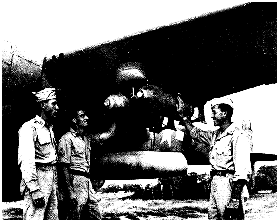
BOMB RACK IN WINGS —The 13th Air Force Service Command in the South Pacific has produced a more versatile and powerful P-38 Lightning plane by designing the external wing bomb rack seen in this official U. S. Air Forces photograph.
