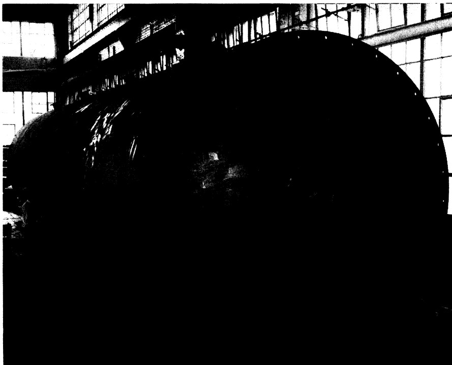
43,000 GALLON TANK —Probably the largest rubber-lined tank, it is used for storing water necessary for the making of high explosives. The rubber lining (work of the United States Rubber Company) keeps the water from coming into contact with any metal.
