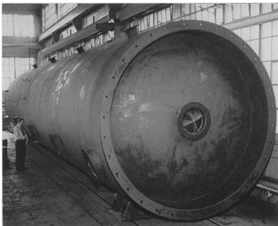
43,000 GALLON TANK —Probably the largest rubber-lined tank, it is used for storing water necessary for the making of high explosives. The rubber lining (work of the United States Rubber Company) keeps the water from coming into contact with any metal.
