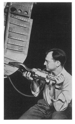
ALLIGATOR-JAWED riveter, operated by compressed air, completely and firmly heads rivets in an airplane frame or in other metal sheet fabrication. This modern air-power tool acts as its own backer up and riveter, and is operated by a single person, as illustrated.
