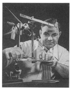
FOR GUIDING SURGEONS' FIN-GERS—This shining steel device locates bullets and other foreign matter imbedded deep in wounded fighting men. A portable field X-ray machine device, shown here being assembled at the Westinghouse X-ray Division, measures the depth and position of the bullet. It also marks the pat'ent's skin to enable the surgeon to position him on the operating table precisely as he was on the X-ray field table close to the combat area.
