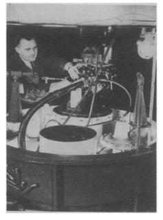
CARBURETORS TESTED—Under simulated flying conditions, this device tests carburetors for Wright Cyclone airplane engines. The hood of the airbox is raised here, with carburetor in place and air and fuel lines attached; when fastened shut, atmospheric conditions at various altitudes can be accurately reproduced. Protecting the tricky operation from fire is the job of the "witches' hats," seen at either side.
