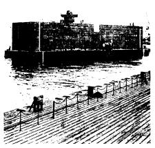
HARBOR PROTECTION — By opening special valves, 146 caissons like the one in this British photograph (above), were sunk into position in the channel for the Normandy invasion. Anti-aircraft guns were placed on the top of most caissons as additional protection of the harbor. These ambulances (left), bring the wounded right up to hospital ships tied at the LST pier head at the British prefabricated harbor on the coast of Normandy.
