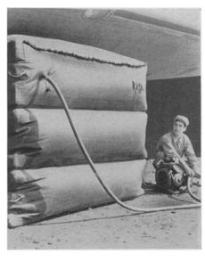
RUBBER PILLOWS, now used to jack up army aircrast on soft ground by filling them with air delivered by a gasoline-driven engine blower, raise the plane without injury to the wings when placed as illustrated in the picture. Each giant bag, when inflated, is six feet high and can support 12 tons.
