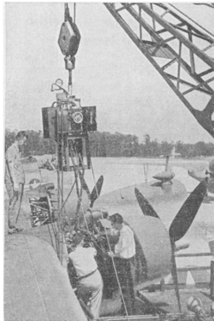
OUTDOOR SPOTWELDING— It is now possible to weld airplane engines on the spot, saving valuable hours. A portable spotwelder was assembled at the Glenn L. Martin Co. to do this job.
