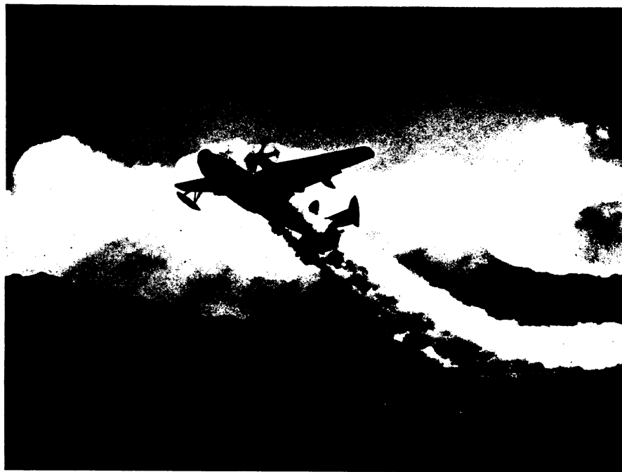
LIKE A SKY ROCKET —Jet-assisted take-off enables the Navy's massive twin-motored Martin Mariner to shoot up from the water rocket-fashion.
