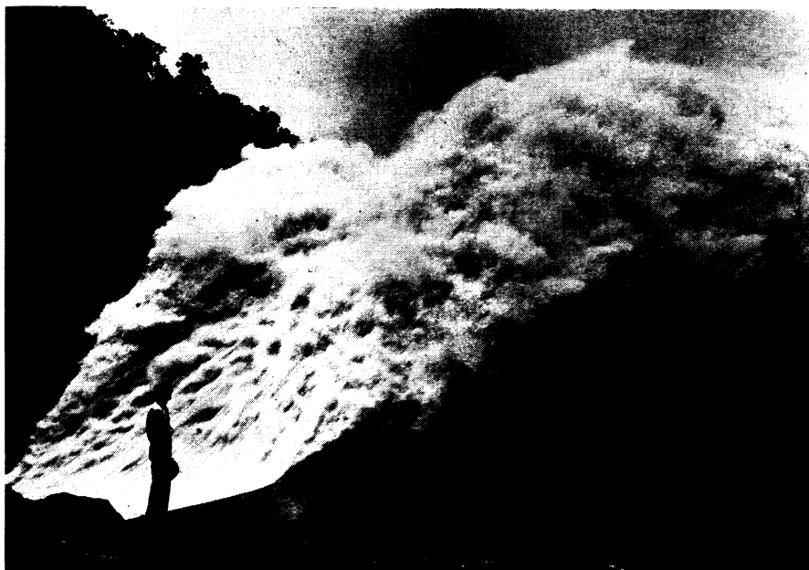
EXCESS POWER —Shooting out from Fontana's spillways, excess waters from Tennessee Valley Authority's newest dam are dispersed into a vast spray to reduce erosion.
