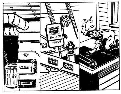
PREVENT FIRES—Home fires could be halved in number if properly constructed and fire-resistant materials were placed at strategic points in the building. Important among the features for fire-safe construction are the heating plant, wiring, and fire-resistant roofing material.
