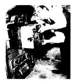
GETS MORE HEAT—With the "down-draft burner," being placed into the firing door of a furnace by Prof. Julian R. Fellows of the University of Illinois, soft coal can be burned without smoke, thus getting more heat from the fuel.
