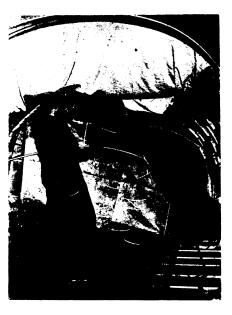
INSURES COMFORT—The cabins of Pennsylvania Central Airlines Capitaliner planes are being lined with down-like glass fiber blankets to protect passengers from both noise and cold. The blankets are similar to those used during the war to provide sound and heat insulation for multimotored bombers.
