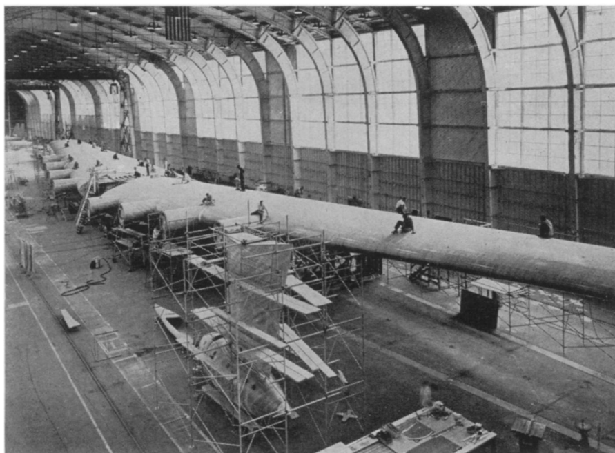
WING SPAN 320 FEET —Some idea of the size of the flying boat may be gained from this view of the wing panels of the H-4. Note the workmen as they appear in comparison with the parts on which they are working.
