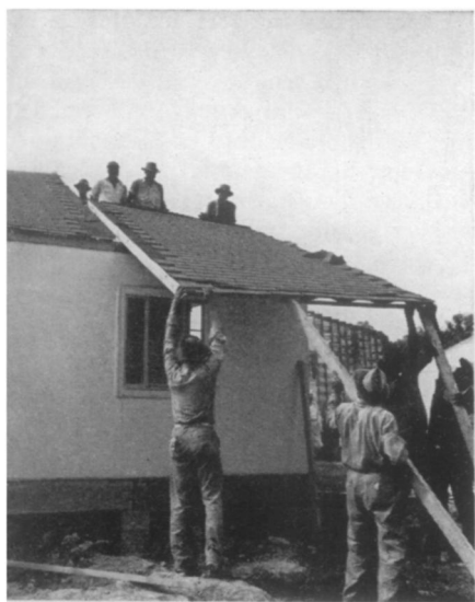
DEMOUNTABLE —Complete roof panels can be placed or removed from a prefabricated demountable house such as the one of the National Housing Agency shown here.
