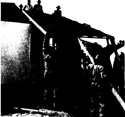
DEMOUNTABLE —Complete roof panels can be placed or removed from a prefabricated demountable house such as the one of the National Housing Agency shown here.
