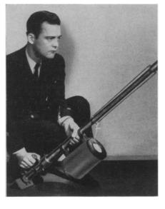
tine-THROWING gun, developed for the U.S. Merchant Marine, for lifesaving, shoots a nylon line 400 yards from the reel shown in the picture. A projectile sometimes used is one with a mechanism for firing a carbon-dioxide cartridge which inflates a float upon impact with the water.
