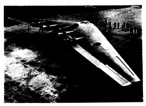
ALL WINGS—Four eight-bladed co-axial propellers, driven by four Pratt and Whitney Wasp Major engines, are expected to push this Northrop Flying Wing XB-35 long-range bomber along at high speed. Wing tip nearest the camera shows one of the wing slots which aid the Flying Wing's efficiency at slow speeds. At high speeds, where the slots are not needed, automatic doors close over them, "streamlining" the smooth surface.
