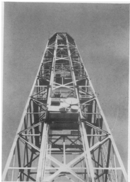
Official U. S. Navy photograph 200 FEET UP—A close-up of the steel tower at Gila Bend showing the elevator with transmitter being hoisted to the top.
