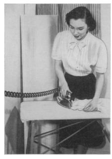
abrasion, tearing and heat from the iron if touched momentarily. The springy cord will stretch six times its retracted length. Science News Letter, June 29, 1946
