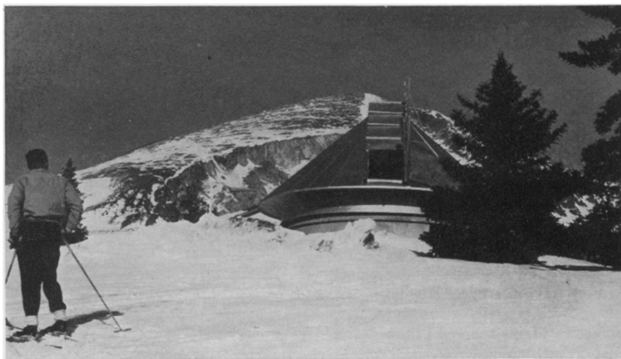
SNOW SLIDE —Dome of High Altitude Observatory, designed specially to study the sun's outer envelope without an eclipse, is shaped to shed snows.
